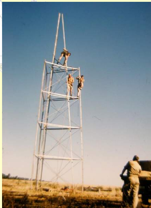
The inner tower frame above the survey mark was for the theodolite and tellurometer and the outer to support the observing platform
