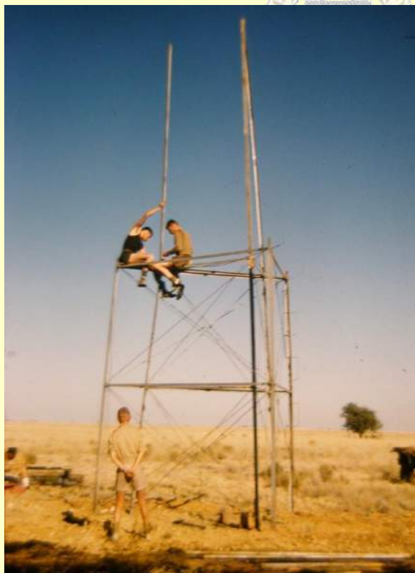
The inner tower frame above the survey mark was for the theodolite and tellurometer and the outer to support the observing platform
