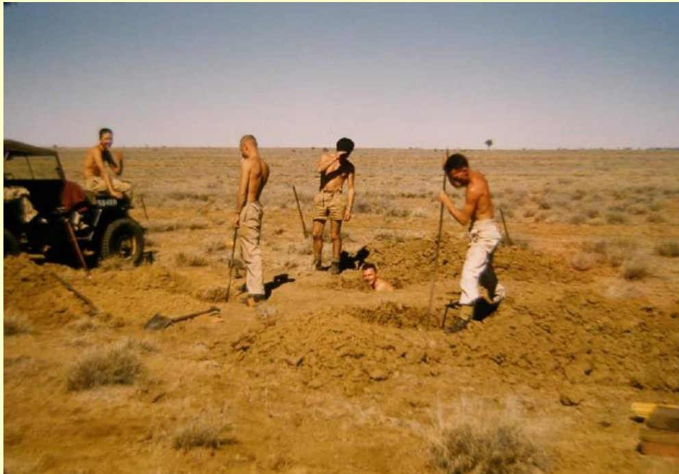
Digging the foundations
