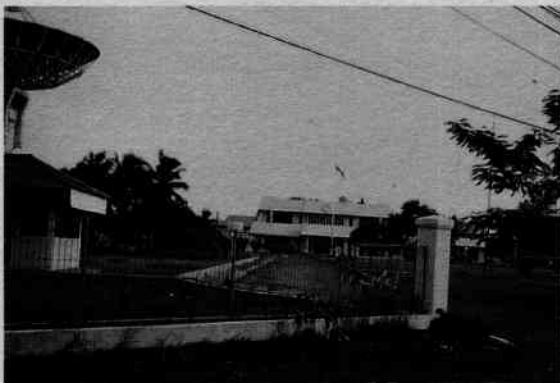
LAPAN Processing Centre, Pekayon, Jakarta.
